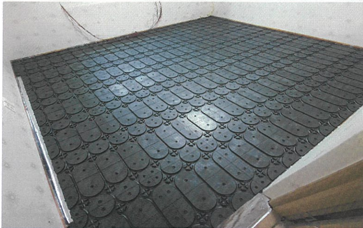
2. Install the panel bottom plates
