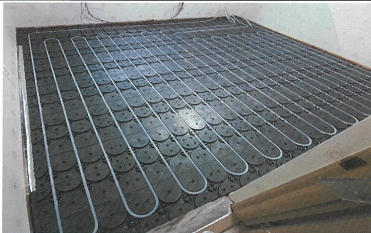
3. Install the heating pipe
